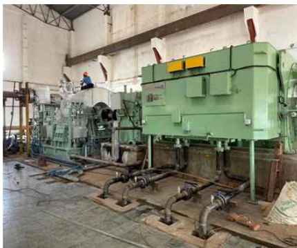
Power House-Turbine, Alternator & Gear box
